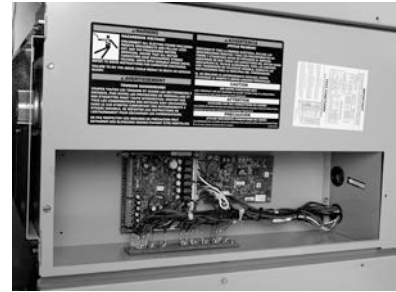
Figure 3. Easy access to terminal board
